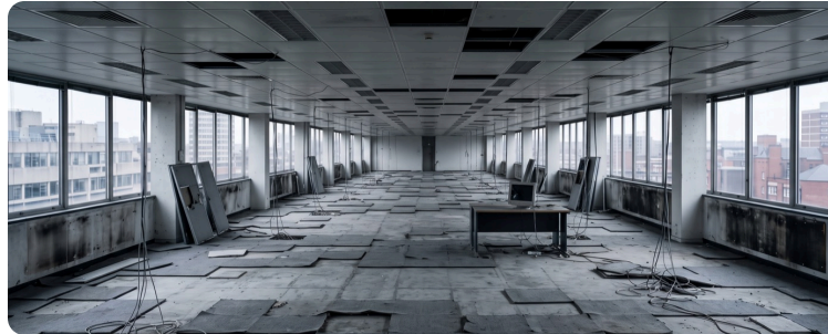
NOW: EMPTY, POWER STILL CONNECTED
